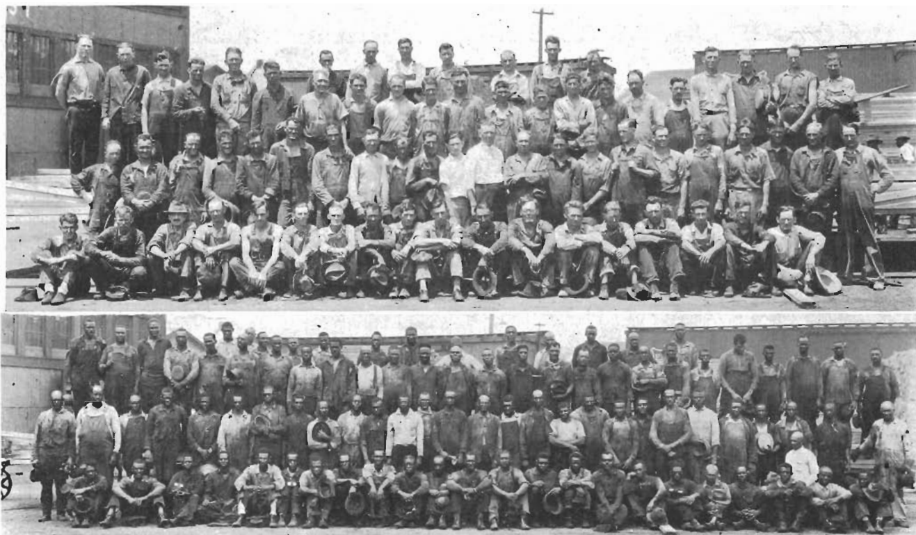
The men in the above two pictures are responsible for the splendid records being made at Yale, Tennessee, in the building of coal cars. Under Jake C. Lutz, car foreman, these workers have set a pace for other roads in swift, efficient car construction. The men in the upper picture are car carpenters and wood mill workers, airbrake men and painters. The negroes in the lower pictures are steel car workers, truck builders and laborers.
