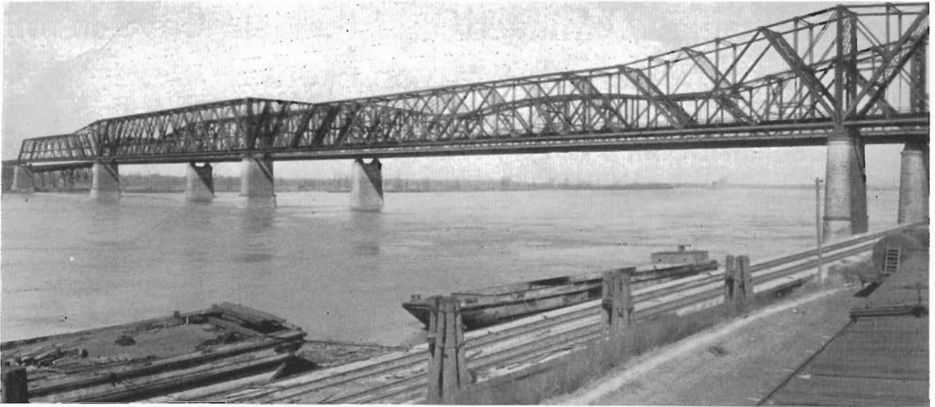
The longest bridge on Frisco rails—the Memphis Bridge—was constructed in 1892 by the Kansas City, Fort Scott & Memphis Railway. The Frisco purchased this road in 1903, and acquired the bridge. Its length, including the steel viaduct of the west approach, is 3,500 feet and the height of its channel spans above high water is 75 feet. Approximately 10,000 tons of steel went into the superstructure.
