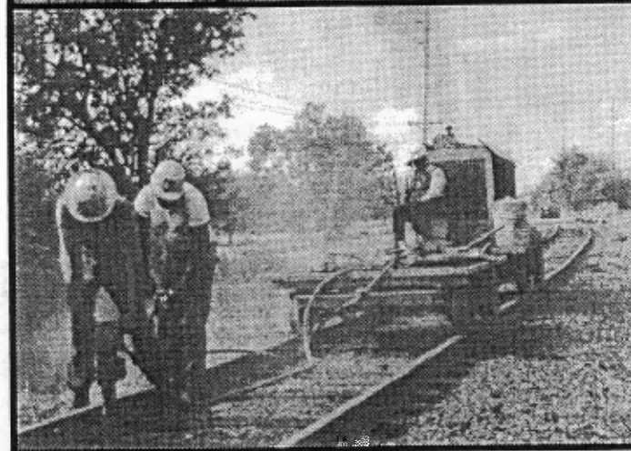
Top: Upgraded rail, new ties and resurfaced ballast between Elm & Walnut St.. Middle: Left side has been upgraded, right side still has the old rail. Lower Left: The Southern Region Rail Gang drives spikes with air hammers using an Ingersoll-Rand compressor. Right: A Jackson Tamper is used to bring the unspiked ties, on the left, up to the base of the rail so spikes can be set. Photos by author. August-September 1976
