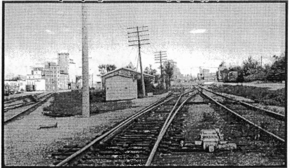
Above: MK Junction looking east to National Avenue in Sept. 1974.
