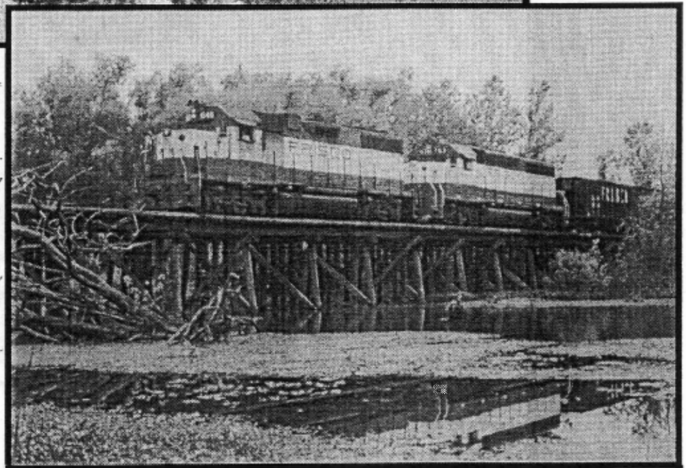
Right: Frisco GP38 #648 & GP35 #763 with an empty coal train on James River Bridge. 6/24/79 Both photos by H. Hall
