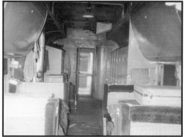
This rare interior photo of ex-Tourist Sleeper 2373, SLSF 105419, shows the upper berth sleeping accommodations still in place. Frisco photo
