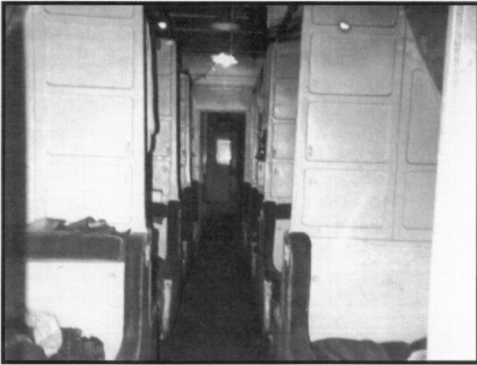
This rare interior photo of ex-Tourist Sleeper 2125, SLSF 105413, shows the individual sleeping compartments still in place. Frisco photo
