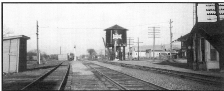
Frisco facility at Billings, MO, March 2, 1948. A. Johnson photo
