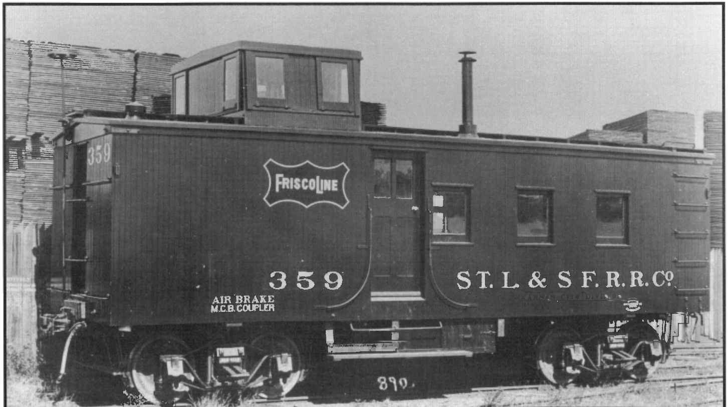
Frisco Line 359 was the last of the second order of new cabooses purchased by the Frisco in 1899-1900. This rare builder's photo was taken at the American Car & Foundry's St. Charles, MO. plant.
