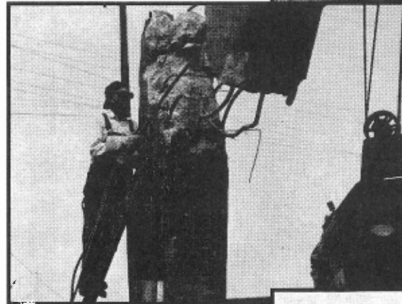
After the first dynamite blast failed, a Terminal Railroad crane held the structure up while the reinforcement rods were cut. Frisco photo
