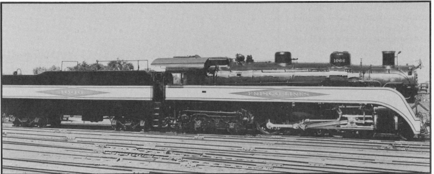
Frisko 1066 was fresh from the paint shop, proudly showing off its new SSP-6 semi-streamlined skirt and paint scheme when this photo was taken at the Springfield North Yards, September 15, 1937.
