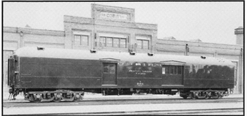
Frisko Baggage/Express series 337-361 (355) as rebuilt by SLSF, Springfield, MO, April 13, 1951. Frisko photo
