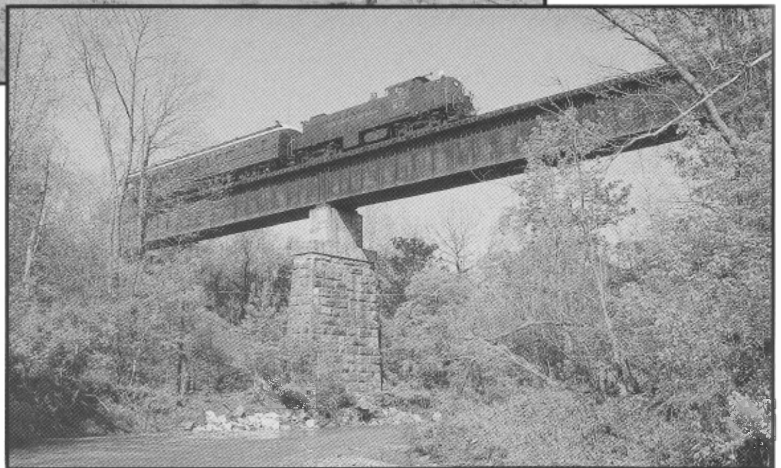
Frisco bridge #325.2, Brightwater Creek, AR, circa. 1990. Arkansas & Missouri Railroad RS1 No. 20 is northbound with Business Car 100. Bob Plough photo
