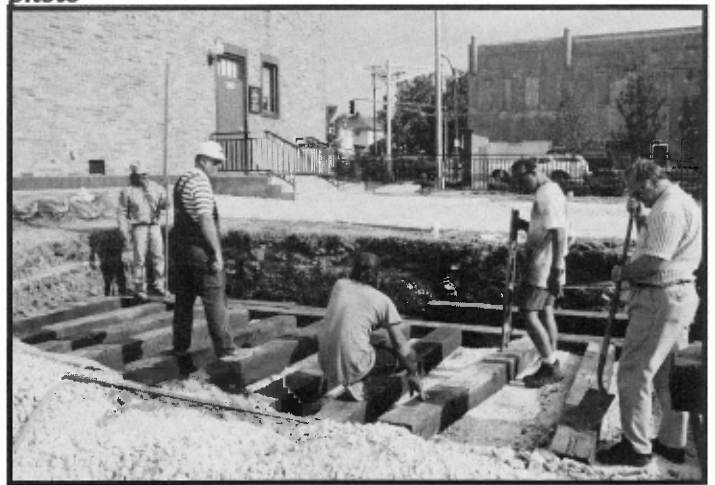
Track work for the final placement of Frisco 1551 was completed by a hard working crew of Frisco Folks volunteers, from left to right: Stan Weddle, Alan Schmitt, Sean Wagner, Jason Justice, and Don Smith.
