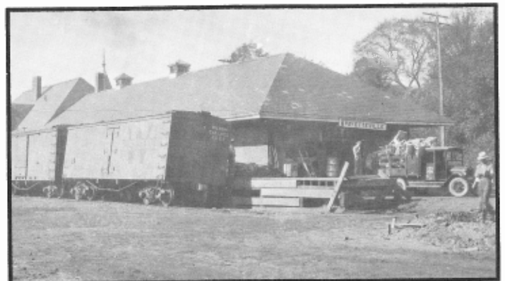
Fayetteville depot, northwest corner, express room dock. Frisco photo
