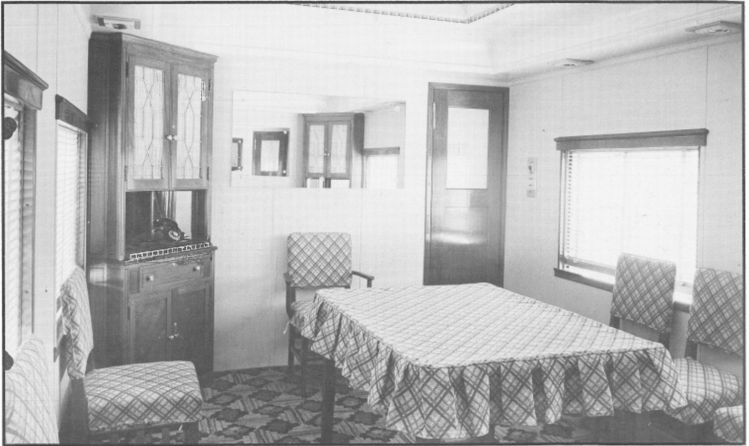
Dining Room looking toward B-end of car, Frisco Business Car Alabama, June 12, 1948, Springfield, MO. Frisco photo
