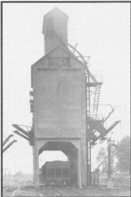
200 ton concrete mechanical coaling plant, Lebanon, MO, October 16, 1942. Frisco photo
