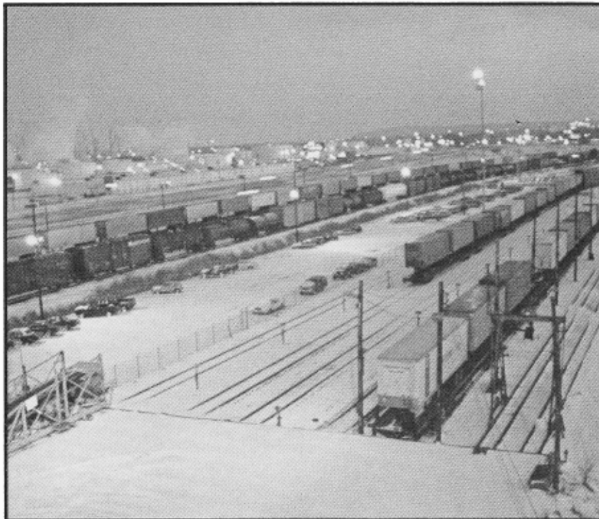
Frisco's Tulsa automobile ramp, still in service in 1978. Frisco photo
