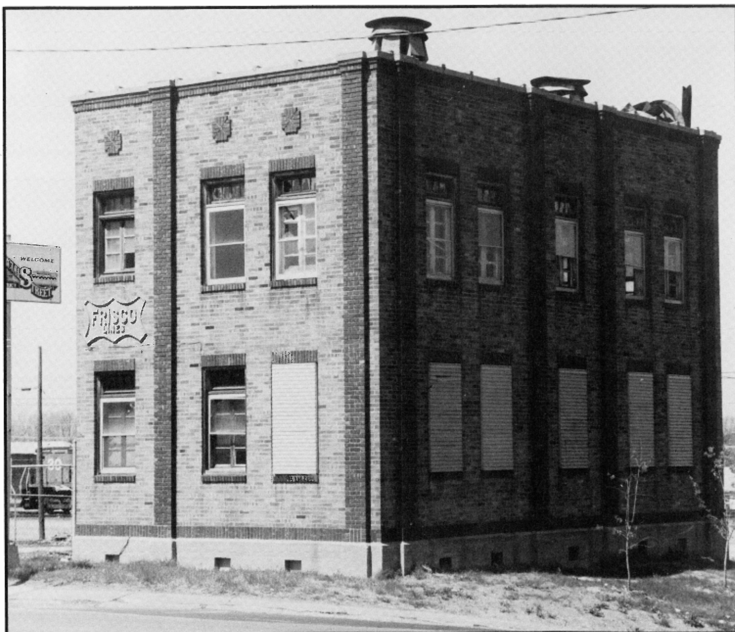
Frisco CTC building, Springfield, MO., built with recycled bricks from the Monett, MO Frisco YMCA, and now the future site of The Frisco Railroad Museum Inc.
