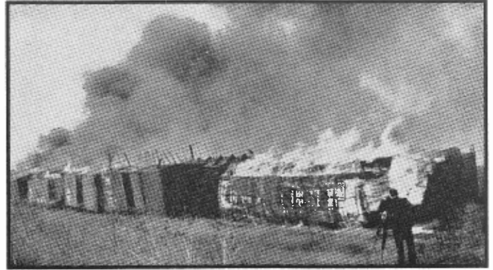
Frisco Box Cars are stacked and burned to remove the wood parts to facilitate cutting the metal into small pieces for handling.
