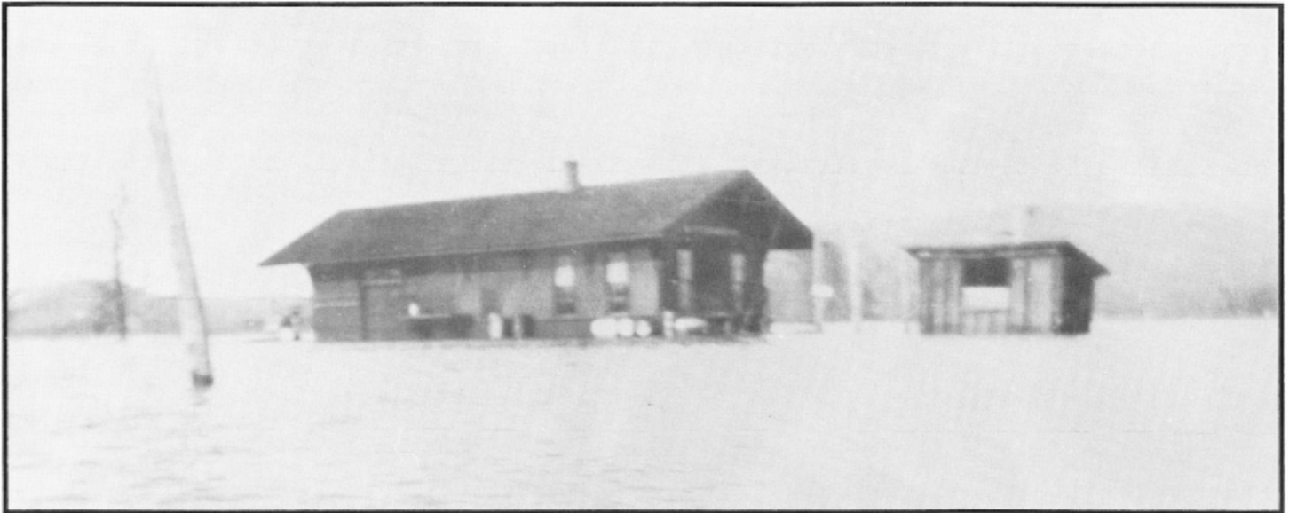
Although the great floods of 1993 put much of the River Division under water, it was nothing new to the folks along the Mississippi River, as witnessed by the rare photo above, showing the Wittenberg depot during an April, 1922, flood. Photo from the collection of Frisco Folk Kevin Johnson.
