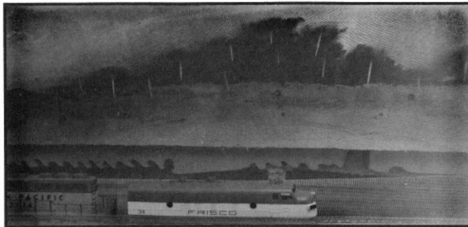
Photo #1, screen wire guard rails
