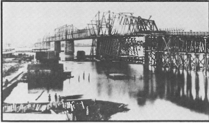
Frisco Bridge construction, 1891, facing west. Michael Finger collection
