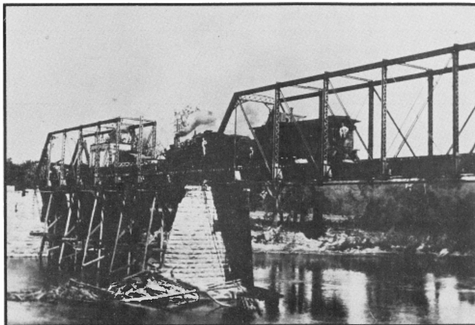
Rare construction photo of Meramec River Bridge, circa. 1889. John Bradbury collection
