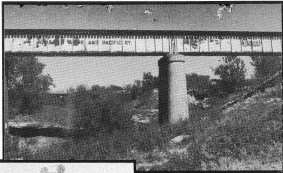
Quanah, Acme, & Pacific Ry. 180', 3 span deck-plate-girder, bridge #728.4, 728 miles southwest of St. Louis, MO, two miles east of Acme, TX, Quanah Sub-Division, Southwest Division. R.E. Napper photo October, 1990
