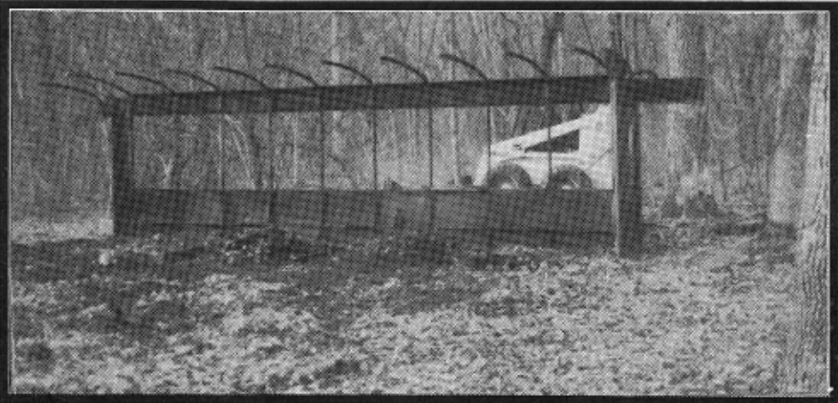
Matt maneuvers equipment to move second half of car.
