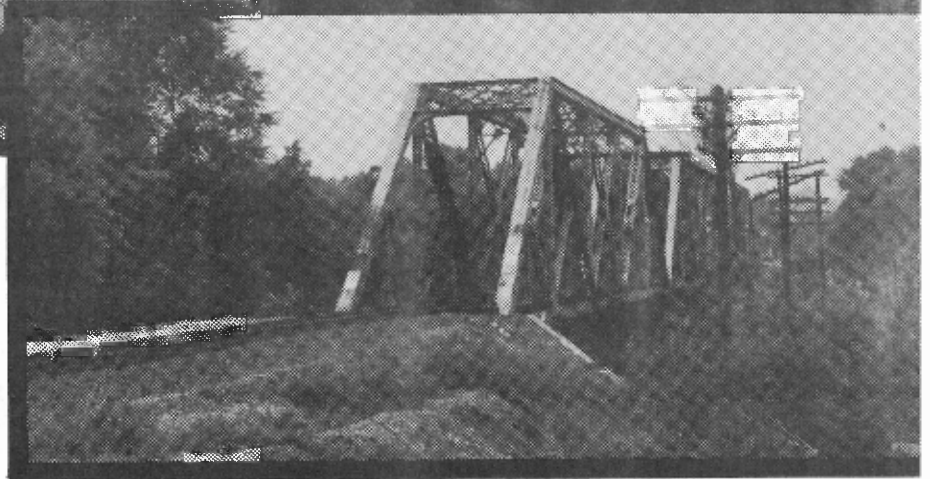
Frisco bridge #18.2 over Meramec River at Valley Park, MO 492', 3 153' through-riveted-truss spans & 1 33' deck-plate-girder span eighteen miles southwest of St. Louis, MO, Eastern Division June 17, 1991 Joe Koch photo
